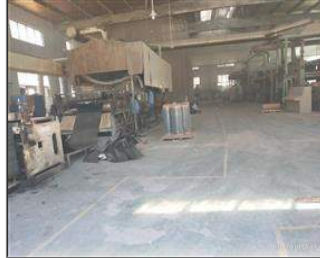
Photo of the inside of the main production hall Calendaring workshop.jpg
