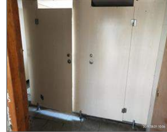
Photo of the sanitary facilities Toilet.jpg
