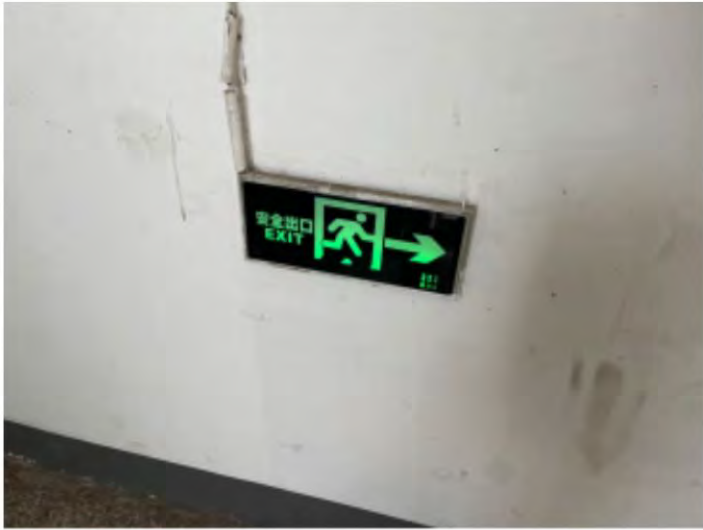
Exit route with marking
