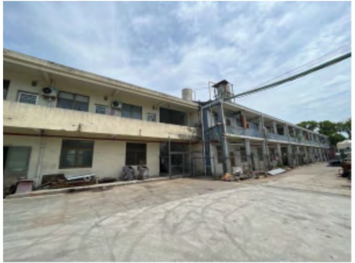
Dormitory and canteen buildings
